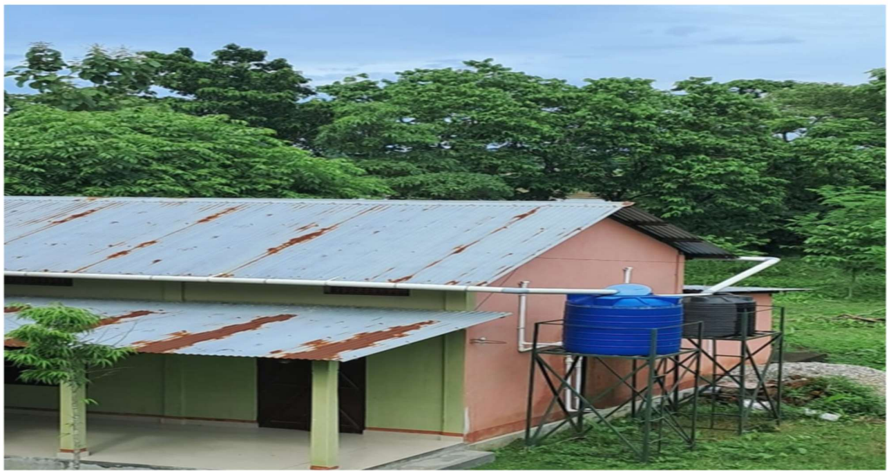
Figure 2 Roof-Top Rain Water Collection
